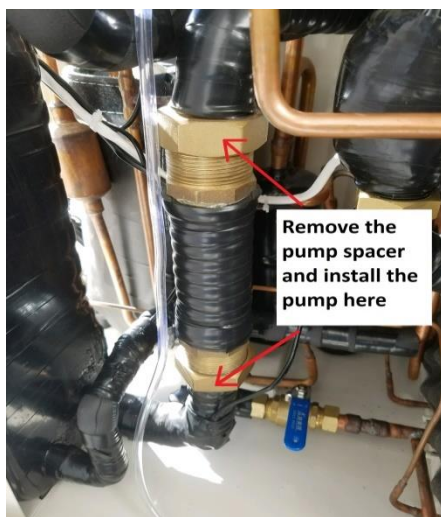
Removing the shipping spacer
